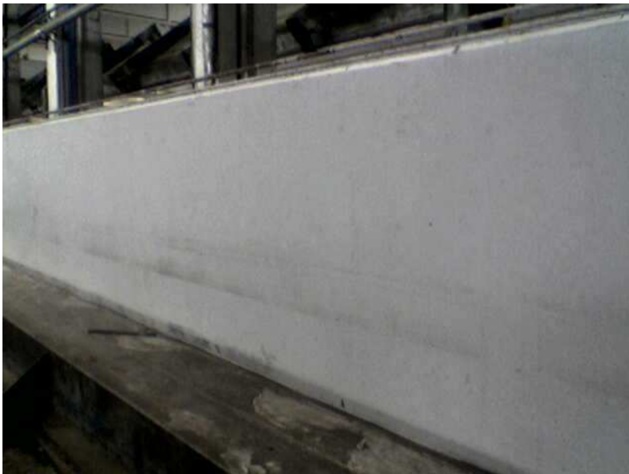
Trave prefabbricata in SCC
